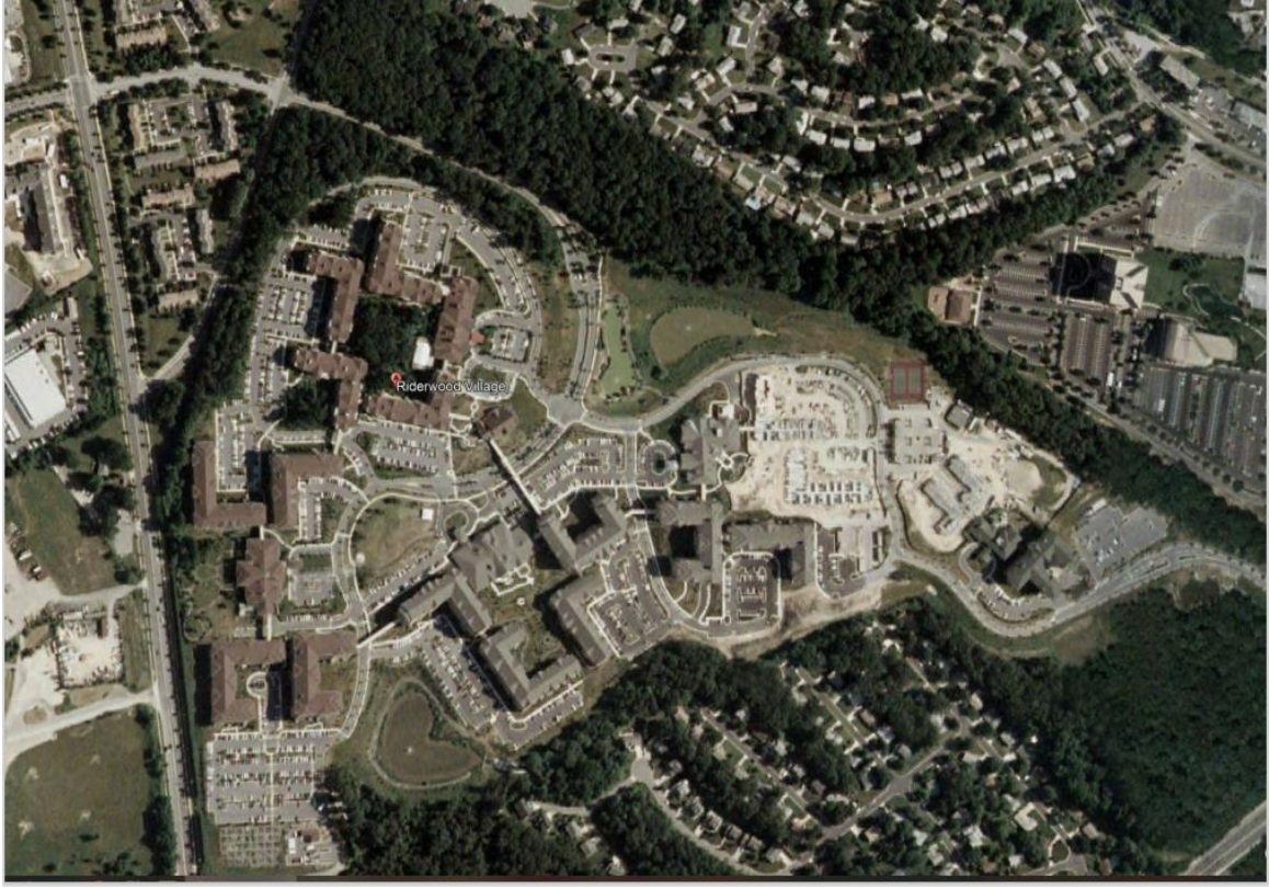
Figure 7. Riderwood Construction in 2005
