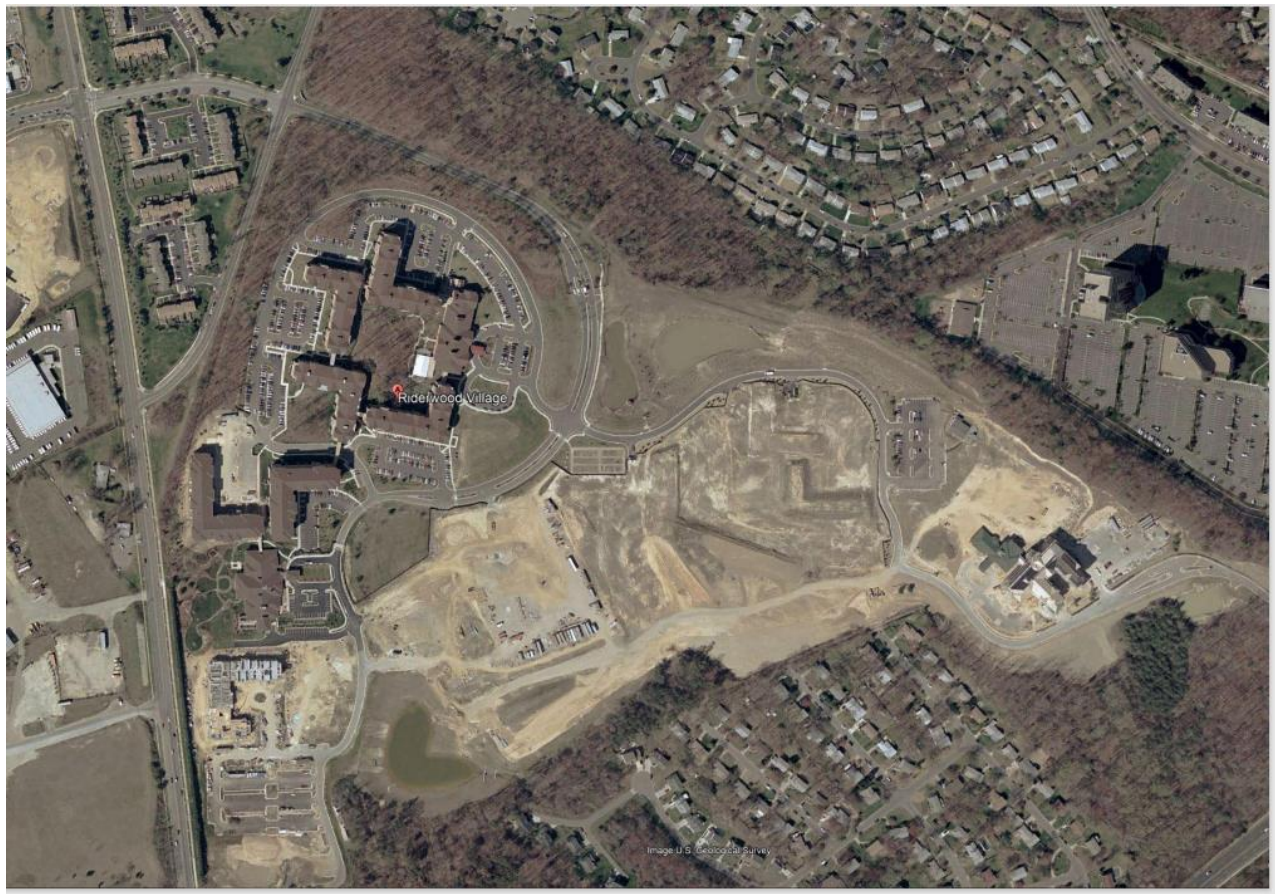
Figure 6. Riderwood Construction in 2004
